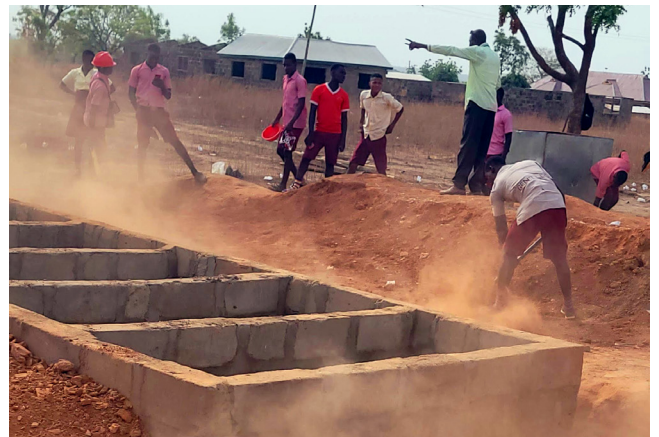
Construction of Walewale toilet block (see also p.18)
